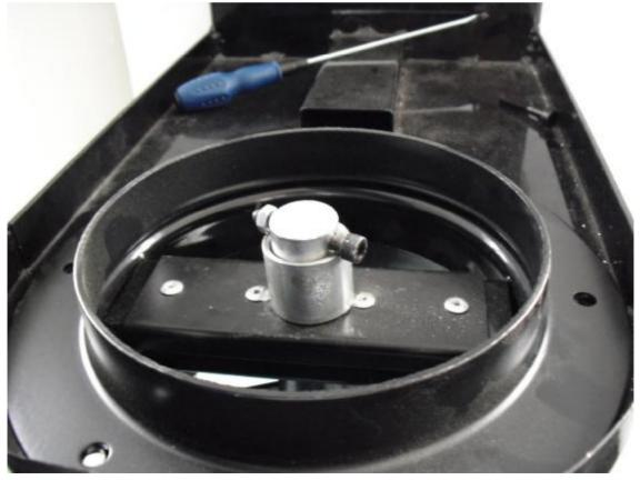
7. Cover the slot between the wall-bracket & flange with the sealing.
