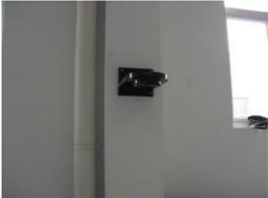
2. Fix the steel flange on the back of wall bracket with 6 bolts.
